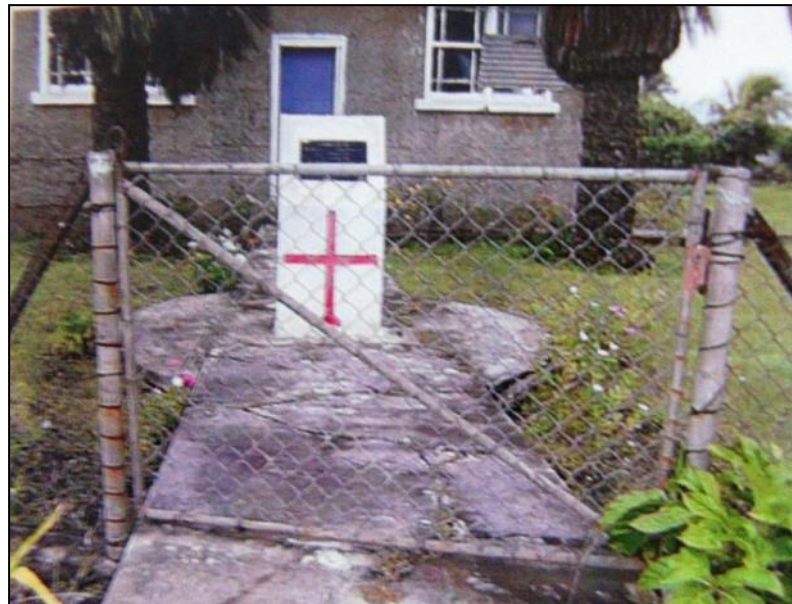
The Anglican Church on the island of Lifuka in the Ha'apai group of Tongan islands has seen better days and is now looking a little worse for wear after weathering many cyclones and earthquakes.
